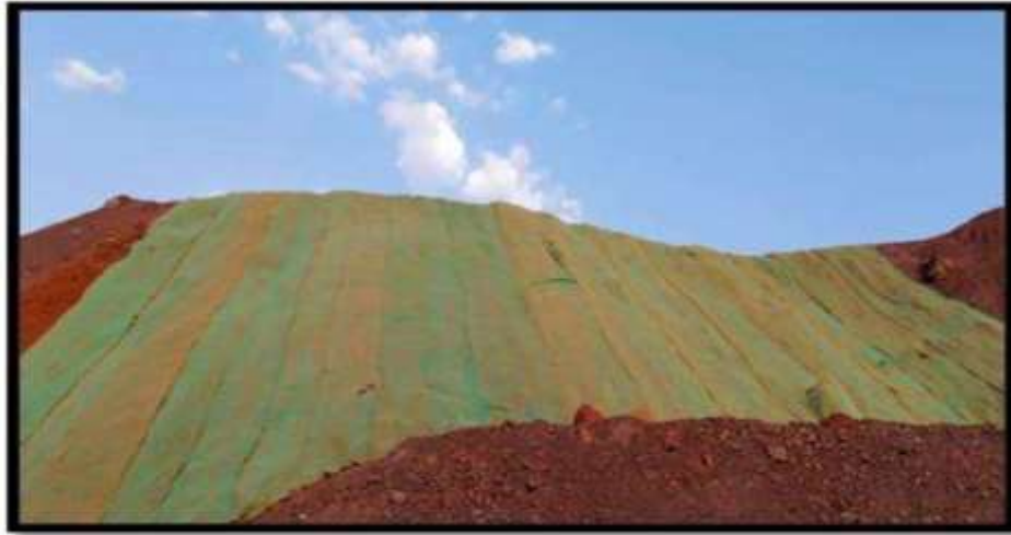
Coir Matts on Dump Slopes
